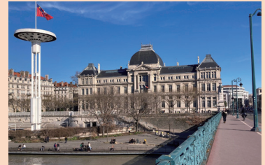
▲The main building of the Jean Moulin University Lyon 3
